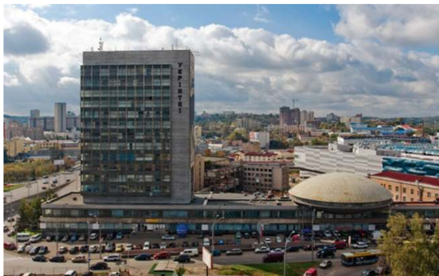
Fig. 20 Kyiv soviet modernism: The “Plate” building, Lybidska Square. (Source: http://kievlast.com.ua , 2016)
